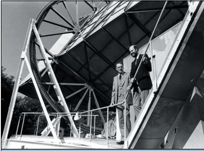
Radio astronomy has helped unravel some of the secrets of the universe. This picture shows the 6 metre horn antenna used by Penzias and Wilson to discover the cosmic background radiation. Their efforts won them the 1978 Nobel Prize in physics.
